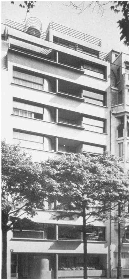
Figure 2. Apartment block, 25 Avenue de Versailles, Paris. Completed in 1931 by Lubetkin and Jean Ginsburg contemporaneously with Villa Savoye, when they were still in their 20s. (Photo Studio Jyska).
